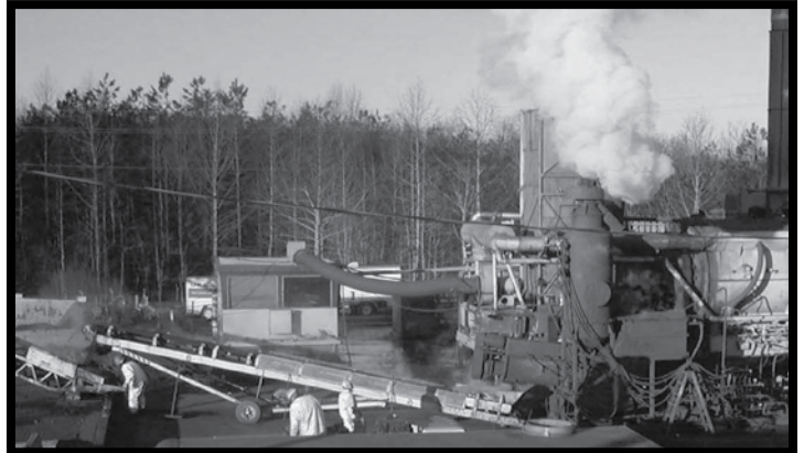
PCB and dioxin contaminated soils were treated with a high capacity indirect thermal desorption unit for the Warren County Landfill cleanup.
